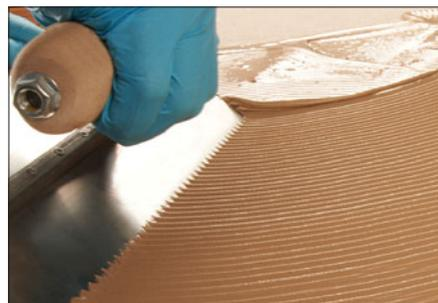
Utilize the V-notched side of the proper trowel to meet the necessary spread rate. While not required, keying or flat-troweling the adhesive onto the concrete could also aid the process and prevent subtle errors.
