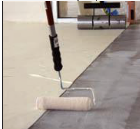
DriTac's latest eco-friendly polyurethane underlayments are part of the company's Total Sound Reduction System.
