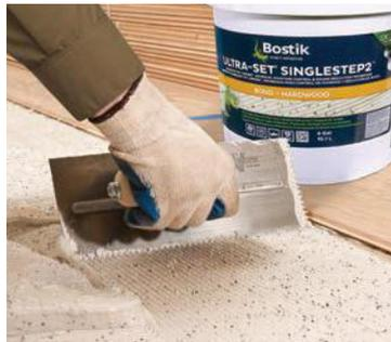
labor, time, material and cost savings, Ultra-Set SingleStep2 features the patent-pending Thickness Control Spacer Technology. This feature can guarantee the proper membrane thickness is maintained between the hardwood flooring and the substrate.
